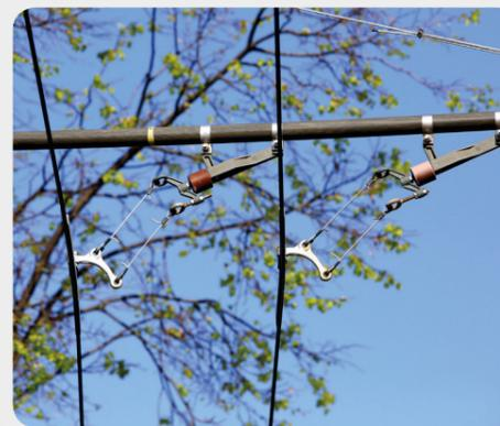
Curve clamps fixed on GRP cantilever
