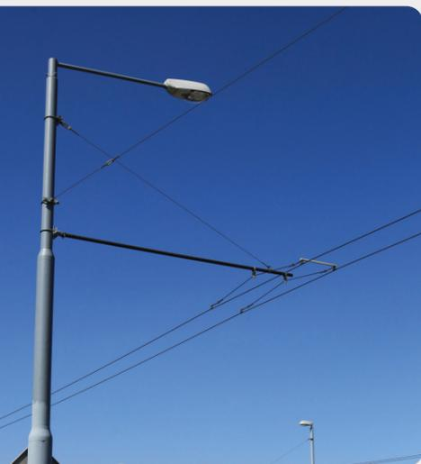
We usually supply GRP (glass-fiber reinforced plastic) cantilevers, but our production includes aluminium cantilevers as well.
