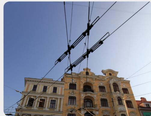
You can choose different geometrical solution ( $20^{\circ}$ - $90^{\circ}$ ) of TBUS x TBUS crossings. Left and right option is available.
