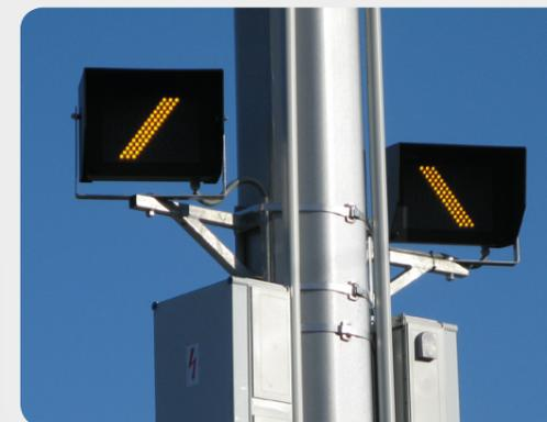
Light signalling informs driver of actual status of switches - direction, blocking and possible incorrect throw over.
