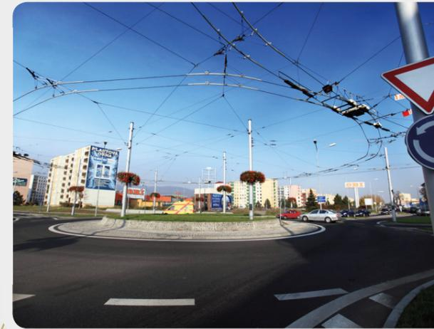
For roundabout solution is suitable use of double switch point controlled by VETRA system with fully automatic operation.
