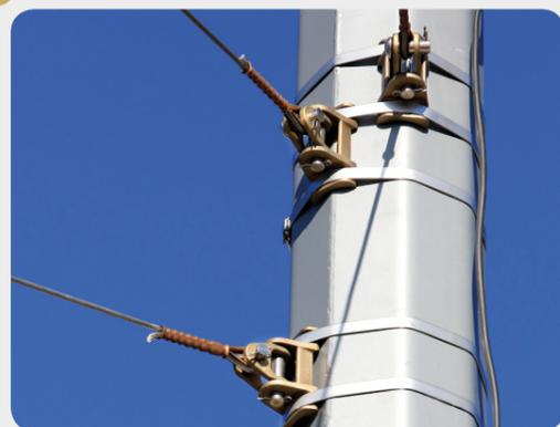
Cross-wire suspensions are fixed to the poles by the various hinge types.
