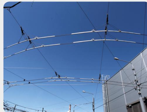
Correct type (length) of used curve clamps has large influence on the operation speed.
